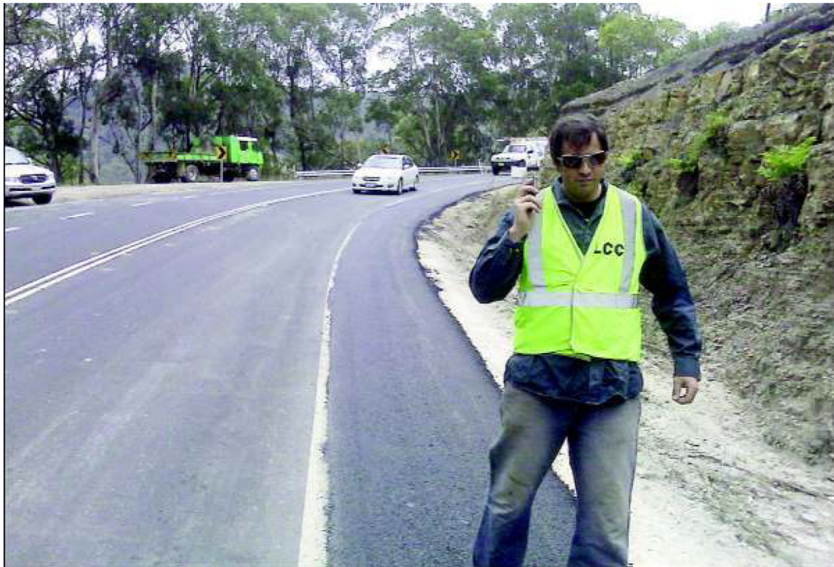
RECORD EFFORT: Joint Managing Director of Sharpe Bros, Richard Sharpe makes an inspection of part of the work along Browns Gap Road
