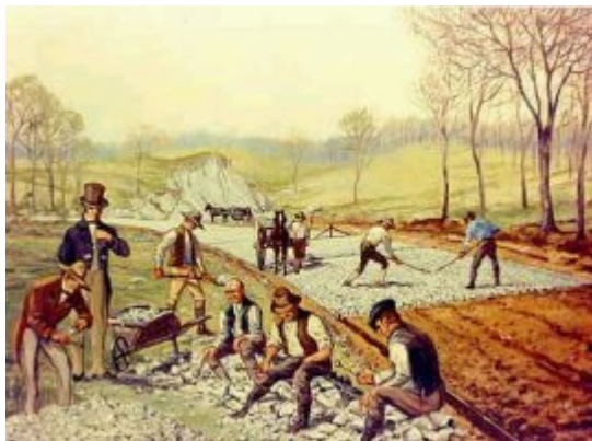
Painting of road work operation
