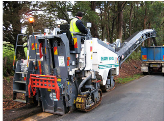
Photo 2 - Profile the road edge to the desired depth.
