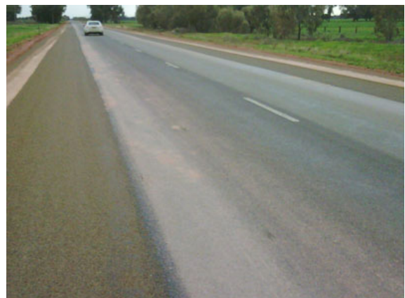
Photo 6 - After sealing the road is wider, safer and stronger.
