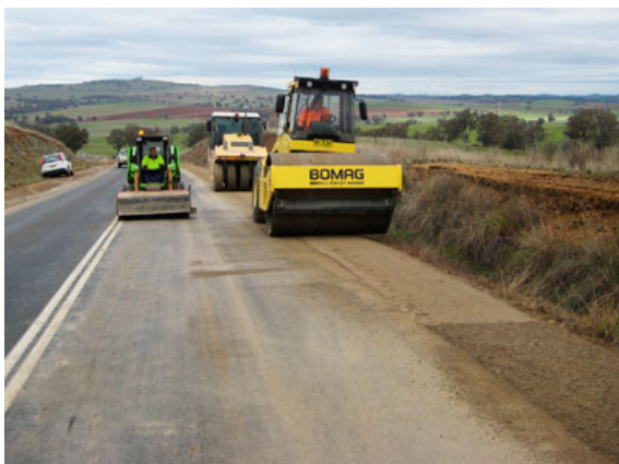
Photo 5 - Rollers follow the Sidewinder. Pave 1 or more layers.
