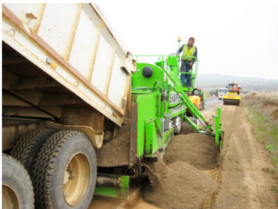
Photo 3 - Pave gravel, road bases or recycled materials.
