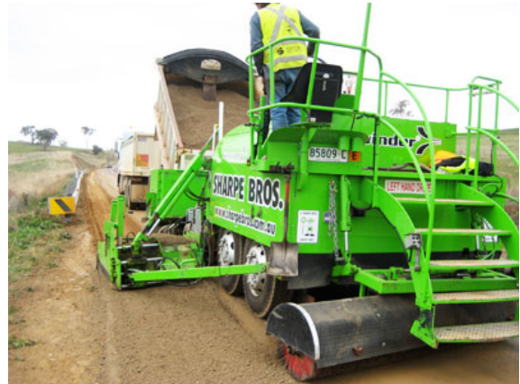
Photo 4 - Pave controlled and consistent layers at 1-3 metres wide.
